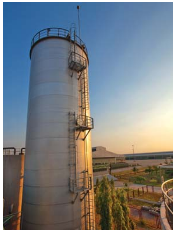
Internal Circulation reactor
