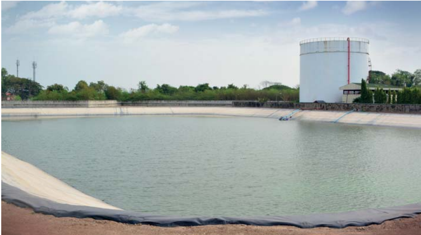
Picture of the reservoir lined with plastic sheets at the Sura Bangyikhan Co., Ltd.
