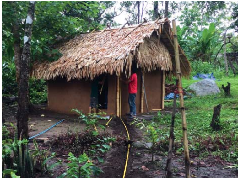
Example of a clay house.
